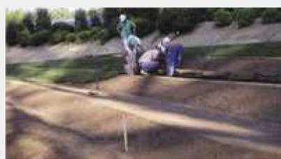
As if traditional turf care doesn’t provide enough challenges, construction of an all-turf amphitheater at Longwood Gardens introduced the added challenge of installing and maintaining grass on vertical surfaces.
